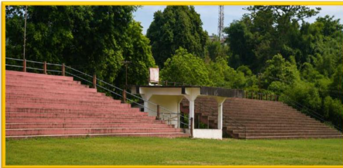
Gallery and Parking Lot
